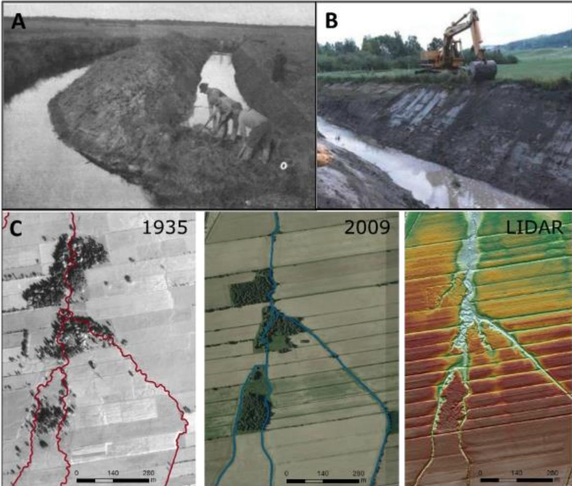
Figure 2: Examples of channelization practices before 1920 A), and after 1930 B), Planform view of the extent of channel straightening commonly found in agricultural areas (here, in the Petite Rivière Pot-au-Beurre watershed) C).
