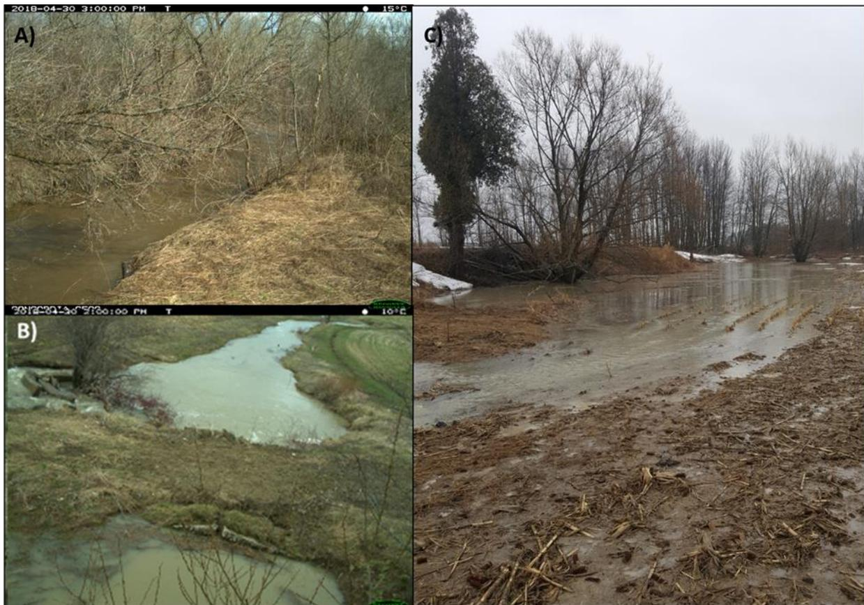
**Figure 79: A) Photo from camera installed at RM facing the ancient meander showing peak fall discharge reaching just below bankfull; B) Photo of narrow culvert at PPauB forcing peak flows to flood surrounding land; C) Example of surface water flooding on agricultural land at PPauB during the spring floods of 2018.**
