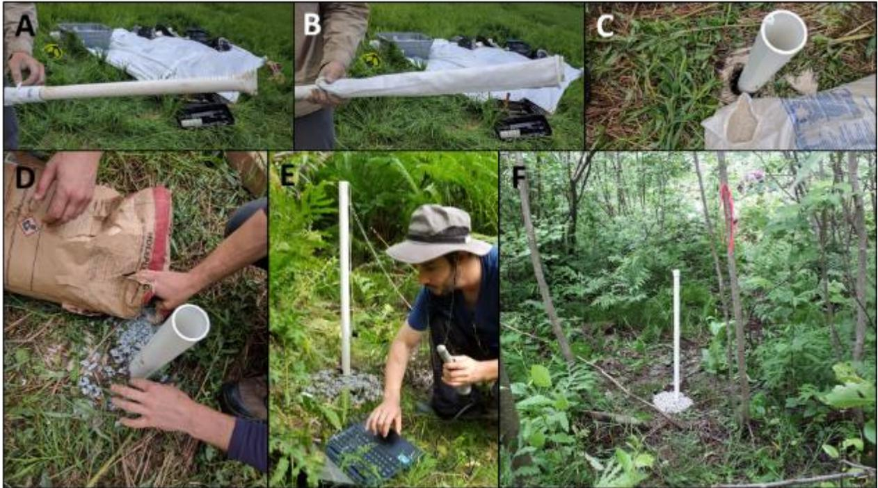
**Figure 30: Example of piezometer installation. Perforated section A), sock used to prevent infiltration of fines B), addition of coarse sand C), bentonite D), logger setup E) and finished installation, P4 at RM mid site F).**
