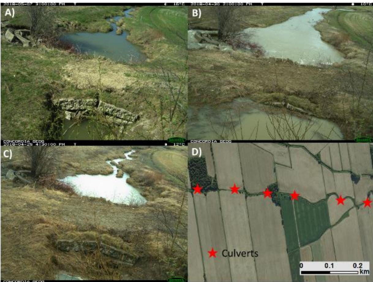
Figure 66: A) Example of a culvert at PPauB at low flow causing a restriction (narrowing) for incoming flow while also contributing to the formation of a relatively deep pool at the outlet of the outlet; B) flow is diverted around culvert at high flow (spring flood) due to its narrow opening; C) debris left over from previous flood further restricts flow through the culvert; D) 6 culverts identified over a 1.5km reach at the PPauB study site.
