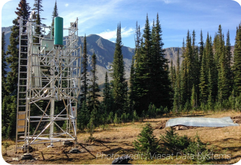
Figure CS10.2 Colpitti Creek monitoring station, British Columbia
